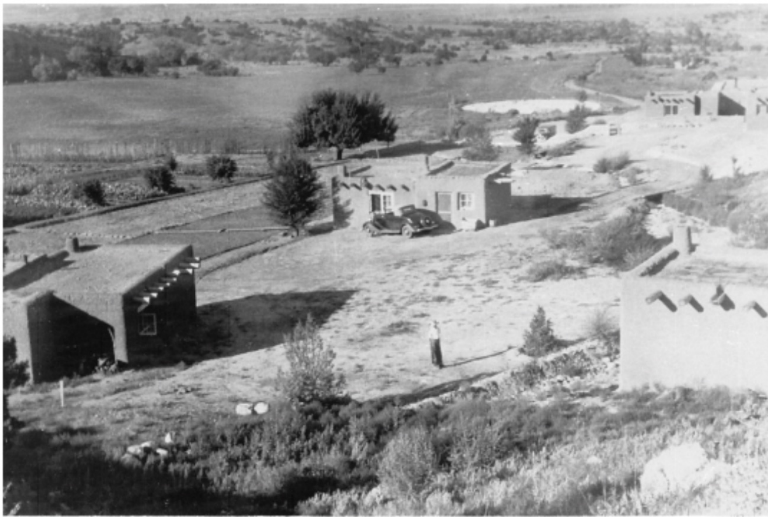
Stanley's crews built the three adobe cottages in the foreground and the headquarters building in the distance. The house to the upper right was built by Arthur Pack and became his home after he left Rancho de los Burros. (Roger H. White, 1935)
